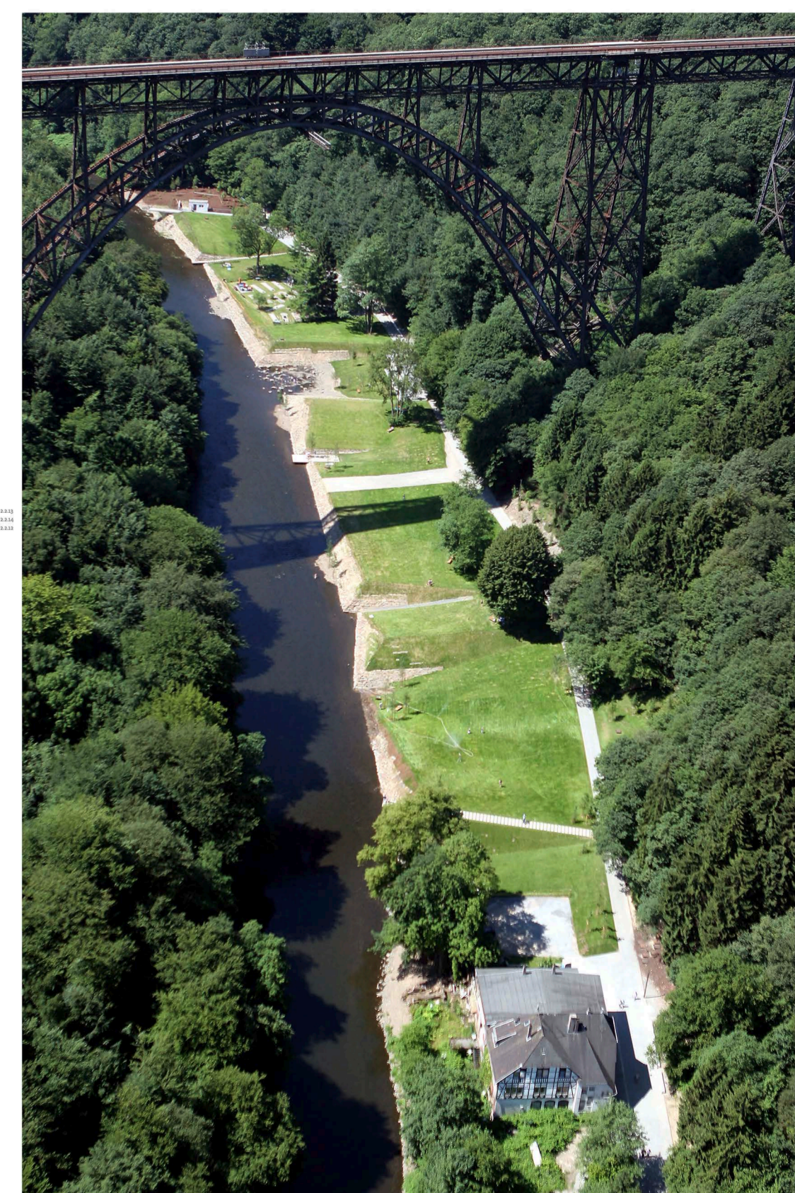
BRIDGE PARK / BRÜCKENPARK
